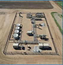
Production facilities are constructed adjacent to the wells to collect and separate the oil, natural gas, and water that are produced. Facility production is 30-45 days of work, completed in stages over about four months.
