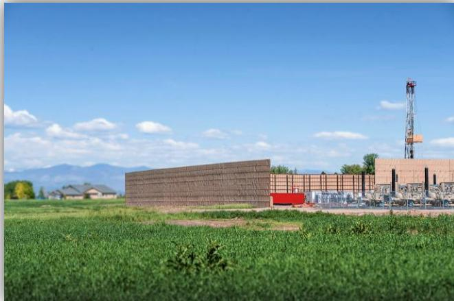
In addition to sound walls, we use upgraded drilling rigs with noise-reducing features and low-noise hydraulic fracturing pump trucks, which are designed to be quieter by using technologies that reduce noise levels without sacrificing operational performance.
