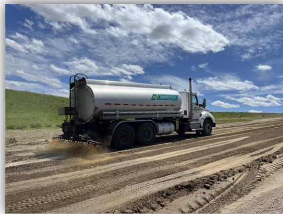
We apply dust suppression to the roads as needed. Various techniques include installing tracking pads and sediment traps, hydro mulching and/or hydroseeding topsoil piles, seeding disturbed soils, and placing and compacting a gravel layer on the working pad surfaces and access roads.
