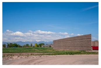
We use upgraded drilling rigs with noise reducing features and quiet hydraulic fracturing technology. These features reduce the noise from our operations. Sound-mitigating walls may be installed on a portion of the site during various times during operations.
