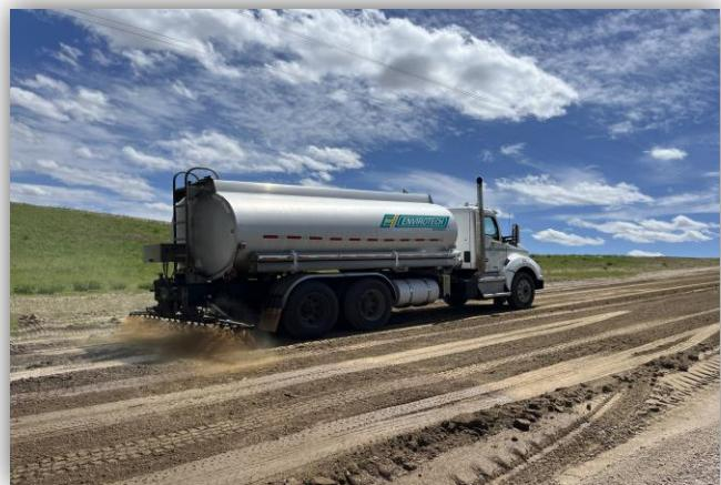
We apply dust suppression to the roads as needed. Various techniques include installing tracking pads and sediment traps, hydro mulching and/or hydroseeding topsoil piles, seeding disturbed soils, and placing and compacting a gravel layer on the working pad surfaces and access roads.
