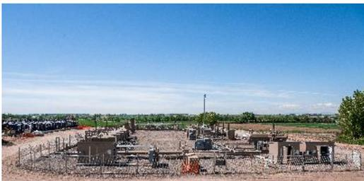
Production facilities are constructed adjacent to the wells to collect and separate the oil, natural gas and water that are produced. Facility production is 30-45 days of work done in stages over a period of about four months.
